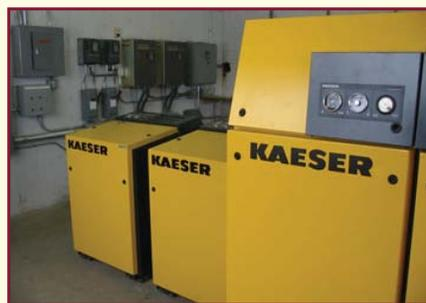
*The goal was to use four rotary blowers to upgrade from the existing gravity-fed system to a controlled pressurized distribution system.*
